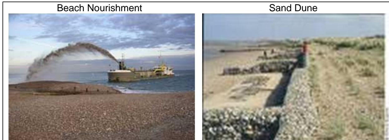
Figure 7. 3 Examples on Beach Nourishment and Dune Stabilization
