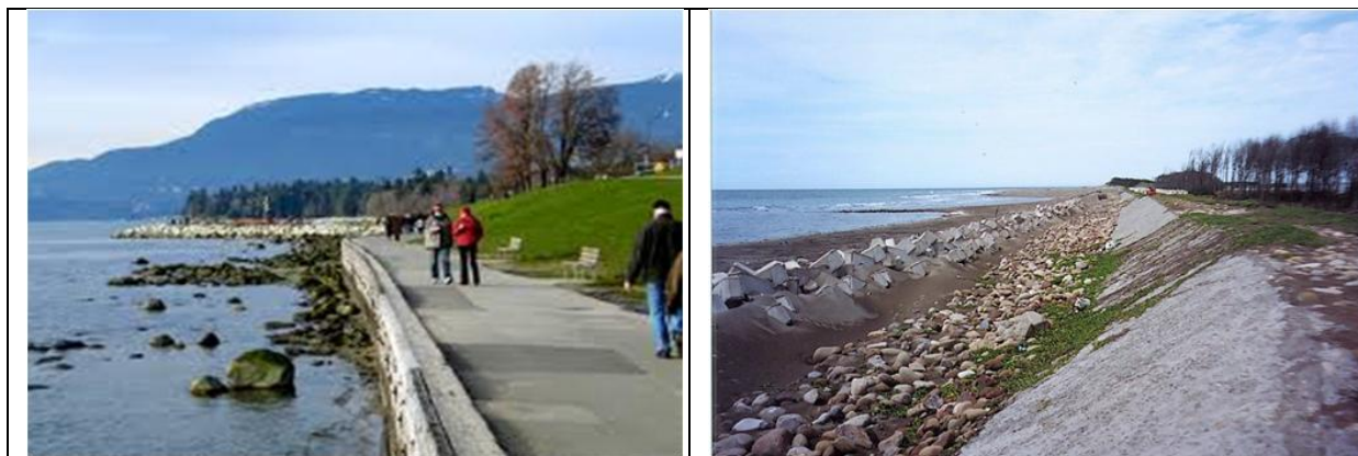
Figure 7.2 Examples on Shoreline Structural Stabilization
