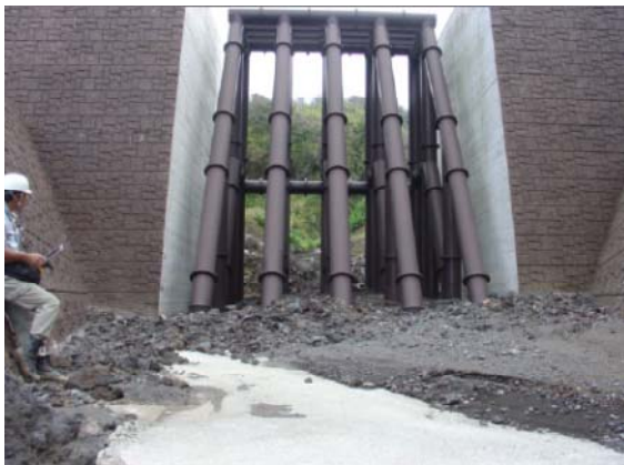
Figure 7. 3 Open type check dam (left) and soft-engineering (right)
