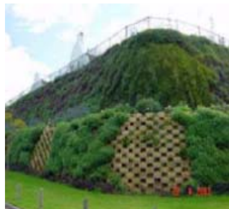
Figure 7. 3 Open type check dam (left) and soft-engineering (right)
