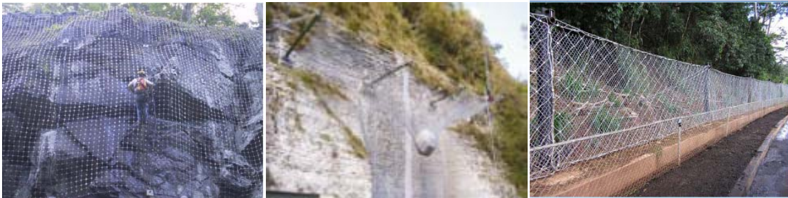
Figure 7. 4 Messing (left), rocks blocks (centre) and boulder fence (rights)
