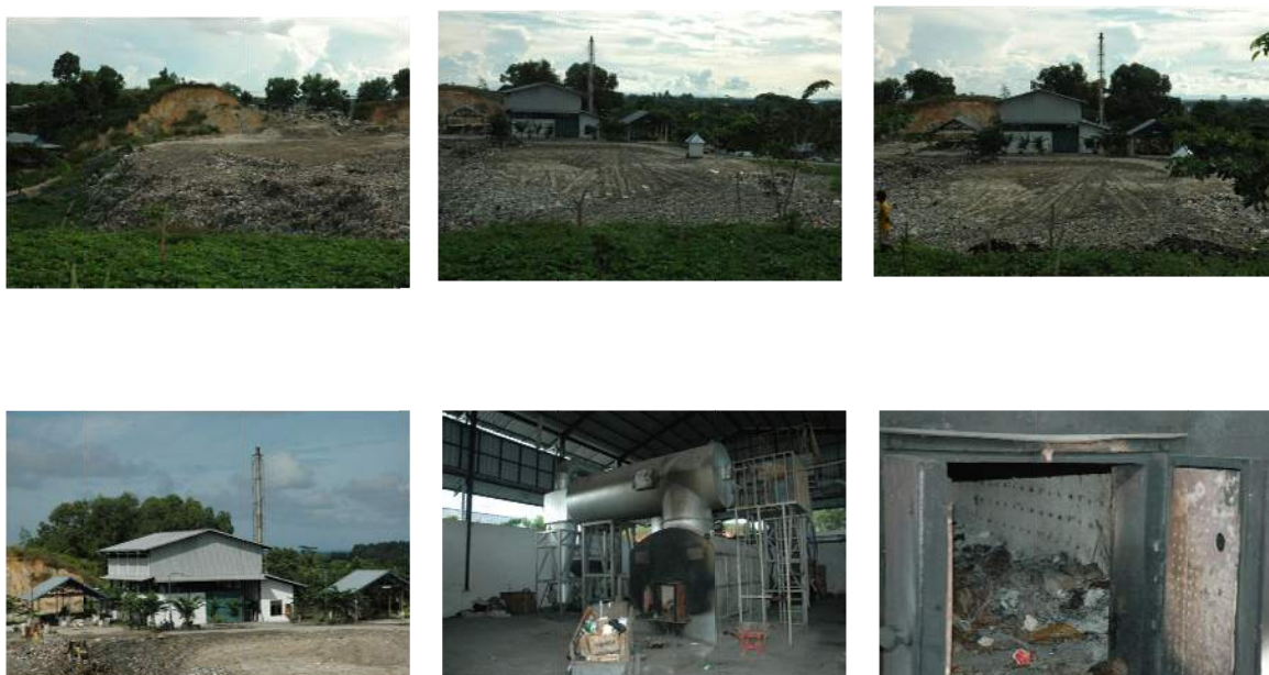
Figure 2-16 Akibabu Sanitary Landfill, Tarakan
